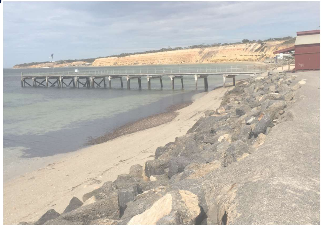
Port Julia Jetty and Revetment
