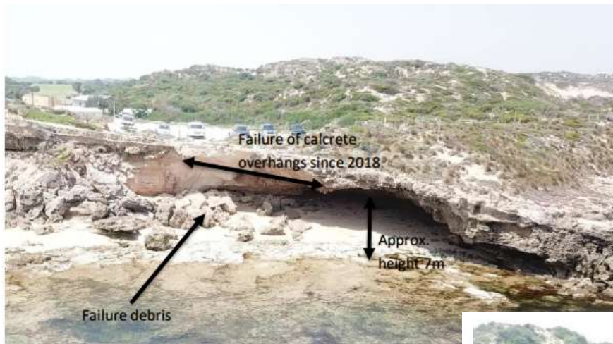
Figure 11: Large undercut cliff at the southern carpark
