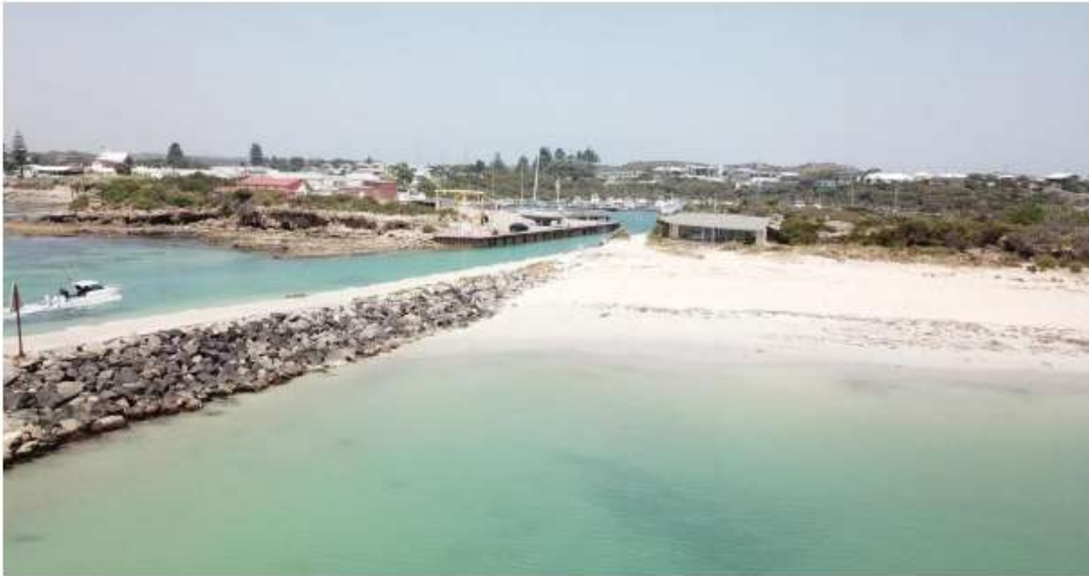
Figure 6: Engineered coastline with a view of the marina breakwater and sheet pile entrance wall
