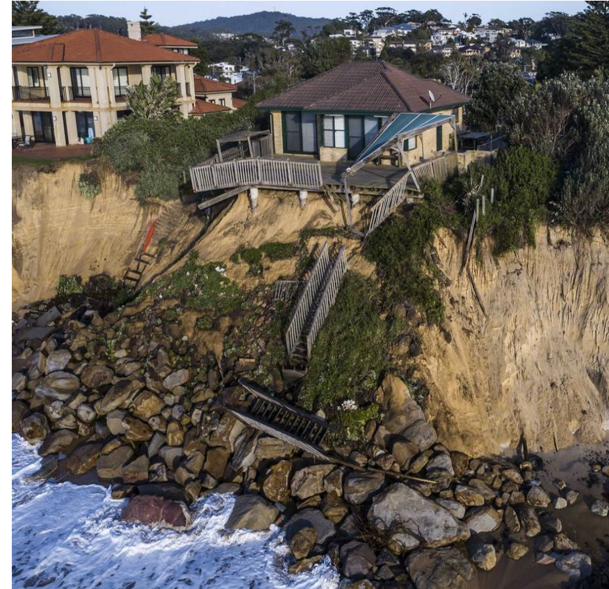
Several beachfront homes at Wamberal (NSW) are in danger of collapsing (NT news 2020).
