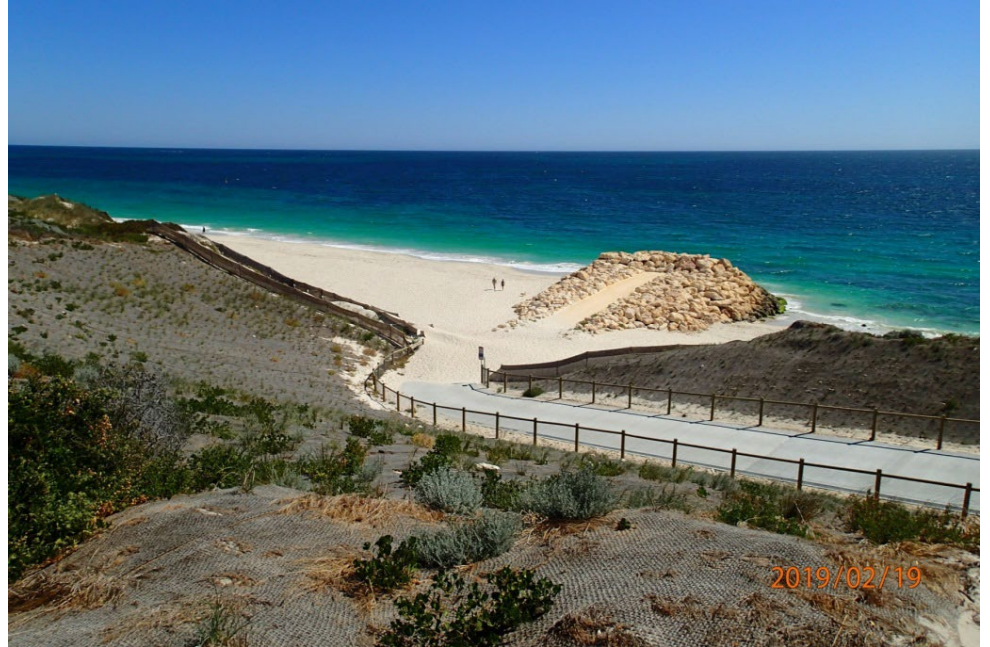
Groyne 4 (new northern groyne)
