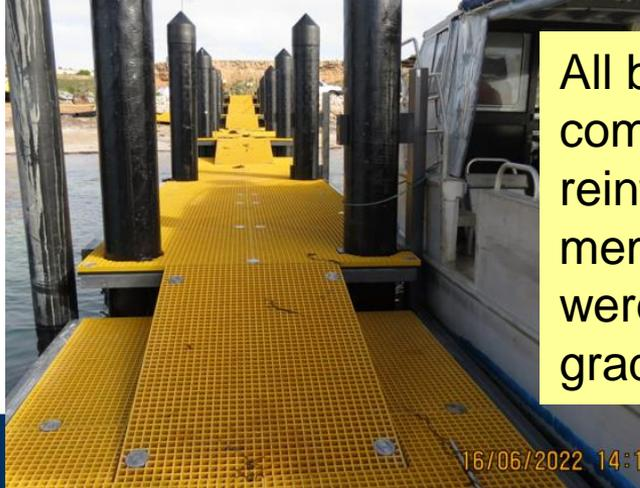
All built from composite fibre reinforced plastic members – only bolts were s/s 316 marine grade
