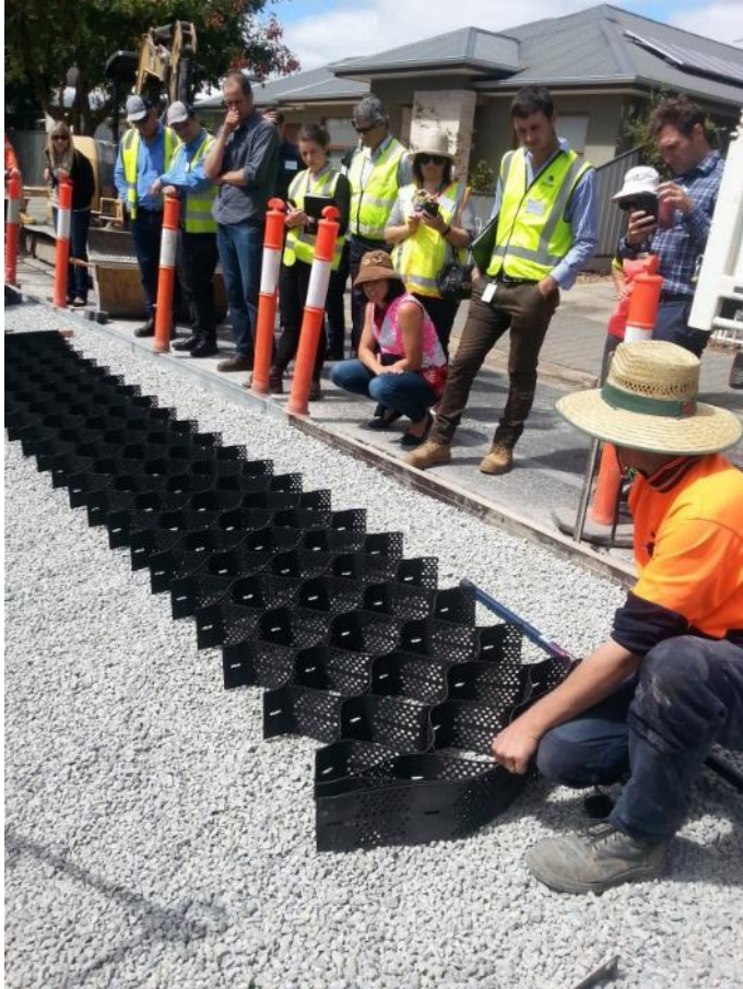
Hillview Road, Netherby – construction of permeable paving. Source: Water Sensitive SA
