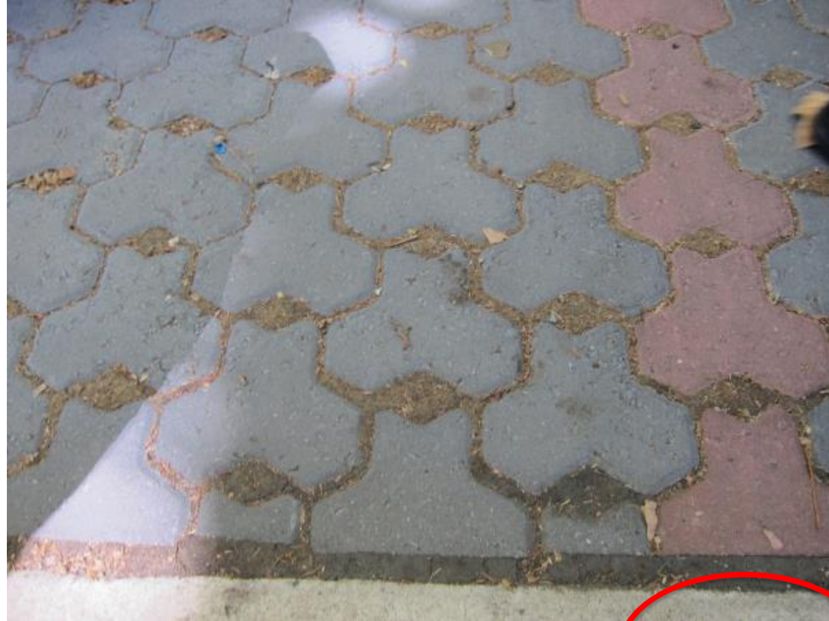
Old Treasury Lane, Adelaide – permeable paving with sediment trapped
